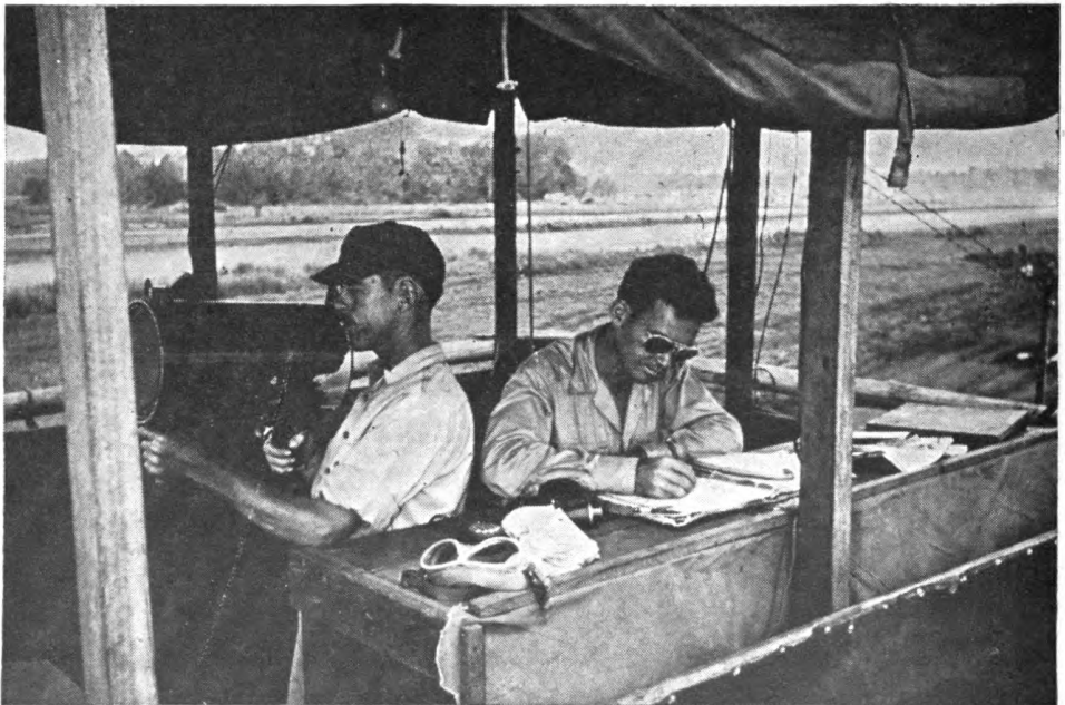
Figure 153. Control tower in operation. Note traffic control lamp.
